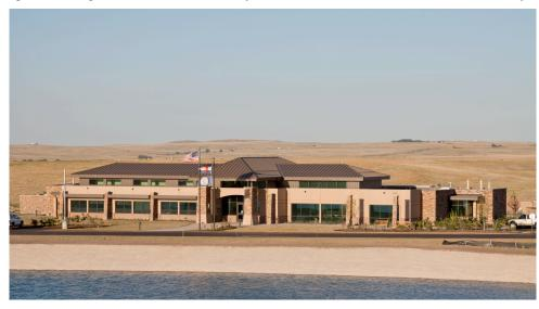
Exterior materials include multi-colored and textured precast concrete; aluminum storefront and windows; synthetic stone facing with precast concrete lintels; and prefinished metal wall and roof panels and copings.
