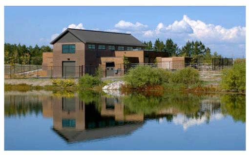
Major materials included split face and ground face masonry units, glass curtainwall, aluminum storefront and metal standing seam roof.
